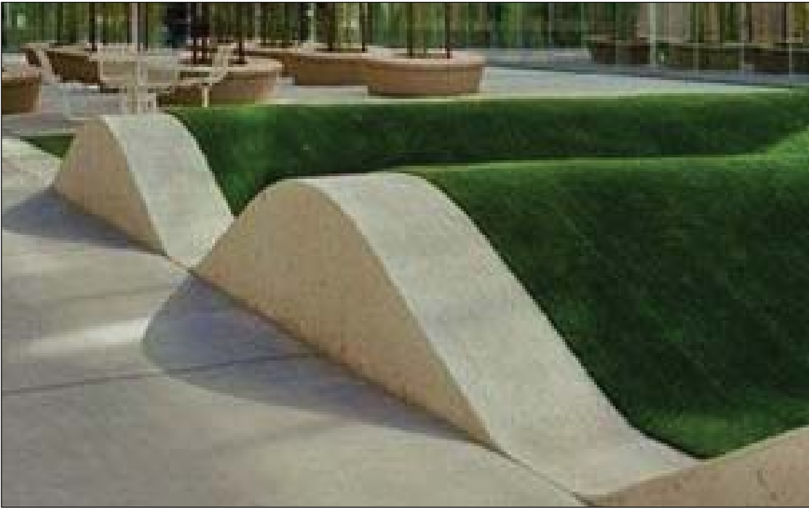
Pre-cast concrete units to form tree planting depth requirements
